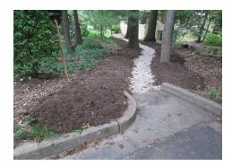
A recent project was the re-direction of water flow from Farsta Court's street drain through a common wooded area. The first part of this proposal included the installation of timber beams and a river rock bed to control runoff and keep it out of neighboring yards. Water will now pass through the rocks, which slows down the flow and disperse the stream as it traverses toward Scandia.
